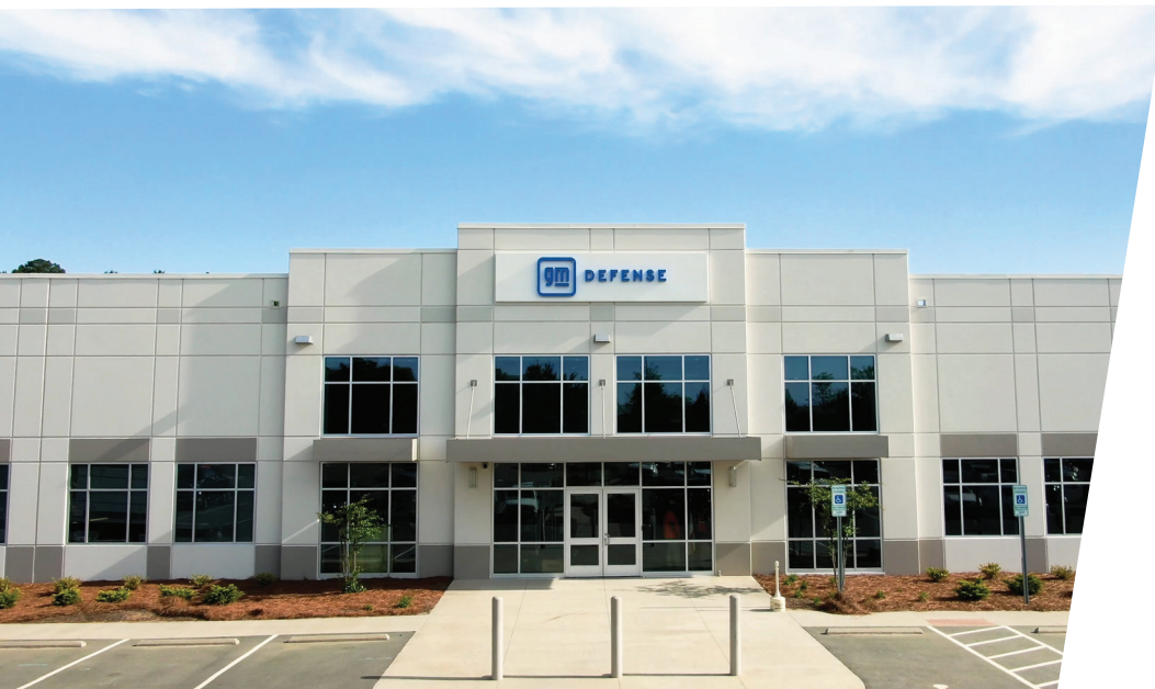
From start of construction to vehicle production, GM Defense stood up its new Concord, NC production facility in just over 90 days.
